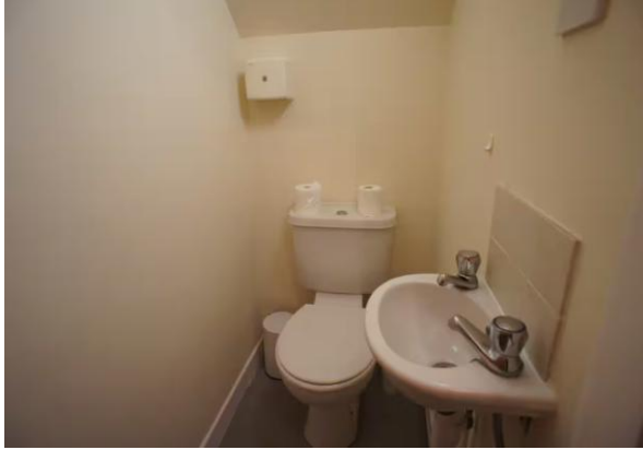
WC – providing a second washroom facility
